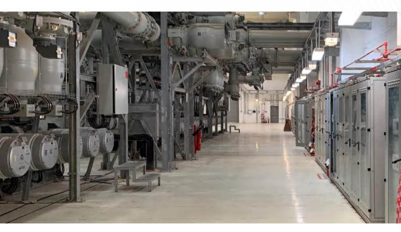
Continuous on-line PD monitoring on GIS using ultra-high frequency (UHF) measurements is an essential part of any electrical condition monitoring program to prevent unplanned outages due to defects in the insulation system of a GIS.
