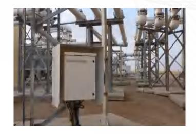
Power Diagnostix's state-of-the-art partial discharge monitoring system was designed based on our GIS expertise and the requirements of our customers. It ensures a continuous and automated analysis of the insulation condition by utilising ultra-high frequency measurement on up to several hundred sensors at frequencies up to some gigahertz.
